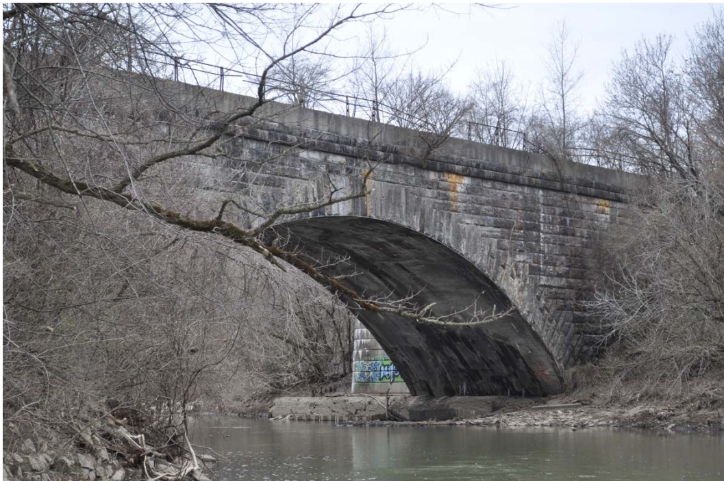
The PRR Panhandle line bridge over Alum Creek east of Columbus.
