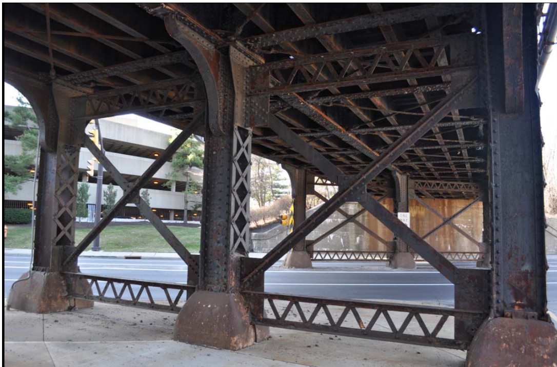
A close up of the PRR Spring Street bridge.
